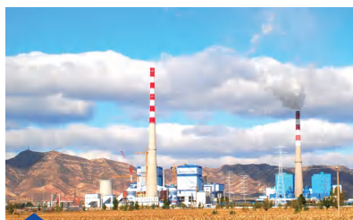
Thermal Power Exhaust Steam Waste Heat Recovery Project
