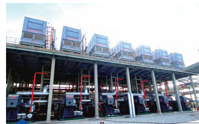
Polycrystalline Silicon Project
