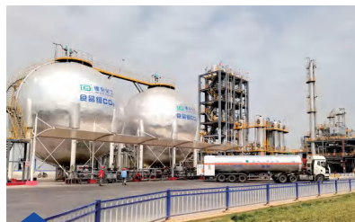
Dehua Chemical CO 2 Liquefaction Project
