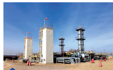
CNPEC Natural Gas Liquefaction Project
